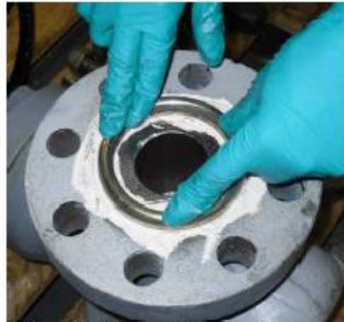
Install the gasket and press to displace the sealant
