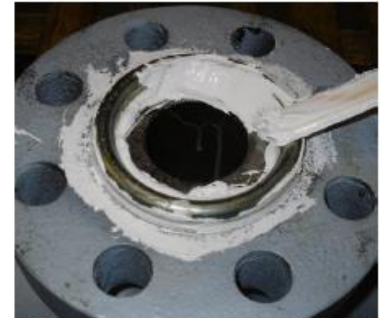
Remove the excess sealant and reposition inside the gasket.
