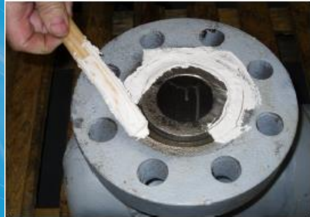
Mix and deploy the Mac-Seal 06
