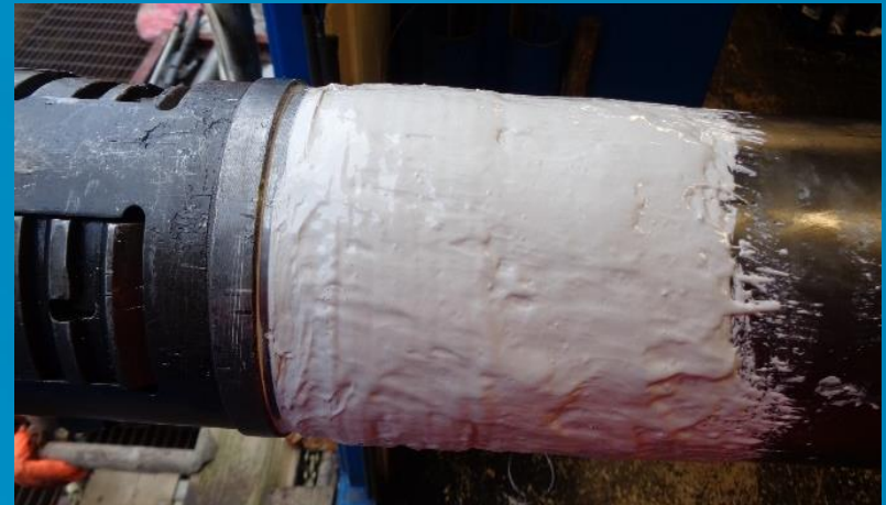
Mac-Seal Applied to WRDHSV at Surface
