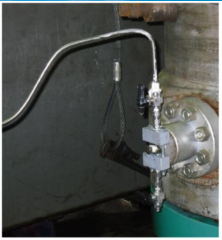
Mac-Seal Injection as a contingency after the deployment of the Mac-Pac
