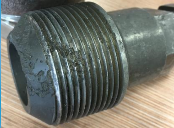
Corroded threads on VR Plug
