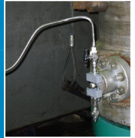
Mac-Seal Injection as a contingency after the deployment of the Mac-Pac
