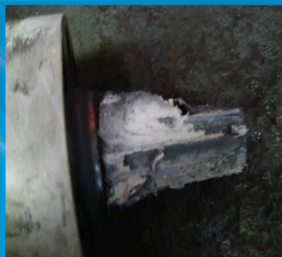
Gate removed with Mac-Pac
